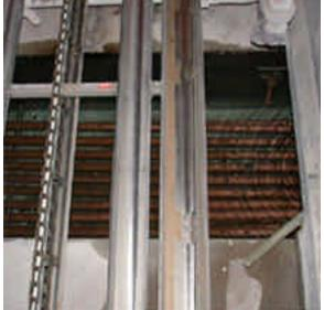
Initial hard deposites on equipment forms within a few days. 60 days after the treatment, scale was wntirely removed and no new scale was deposited.
